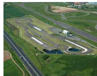
Driving Safety Centre
